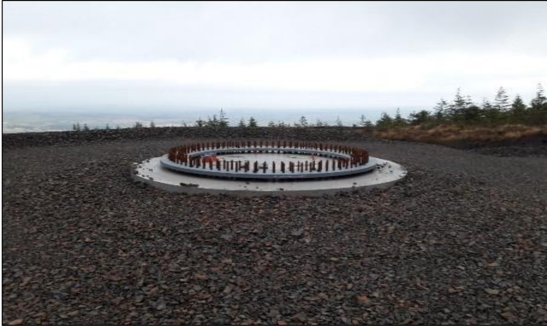
Plate 3-4 Turbine Foundation Back-fill Complete
