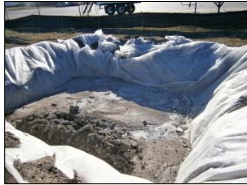
Plate 3.2 Concrete washout area
