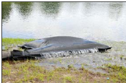
Plate 4.1 Silt Bag with water being pumped through
