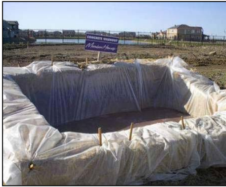
Plate 3.1 Concrete washout area
