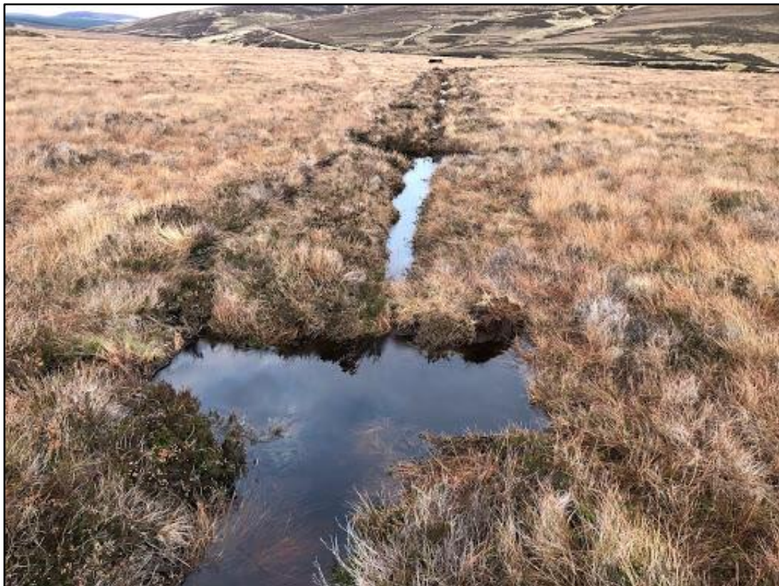
Plate 2.4 Example of peat dams to be used for on-site drain blocking.
