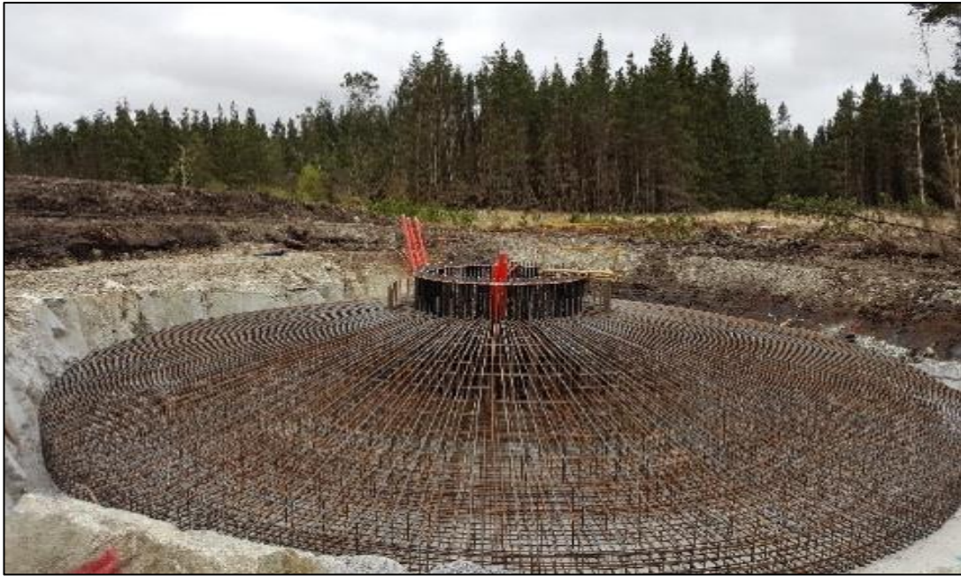
Plate 3-2 Turbine Base 'Anchor Cage'
