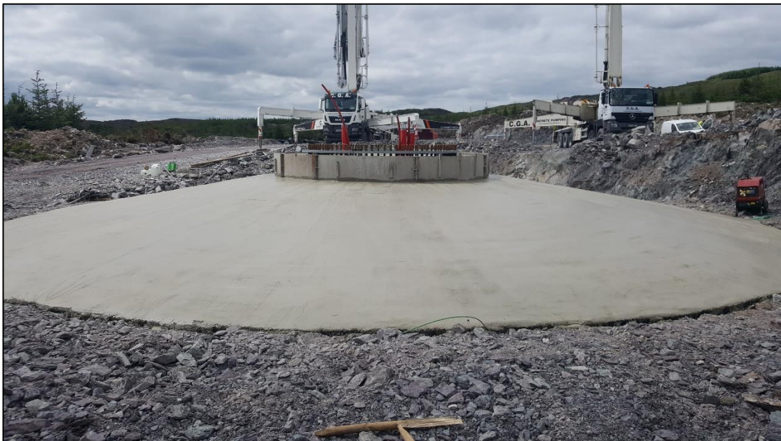
Plate 3-3 Turbine Foundation Poured
