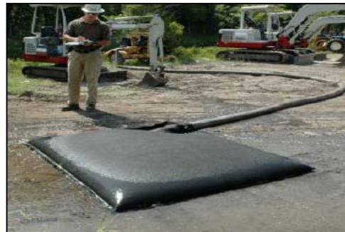
Plate 4.2 Silt bag under inspection
