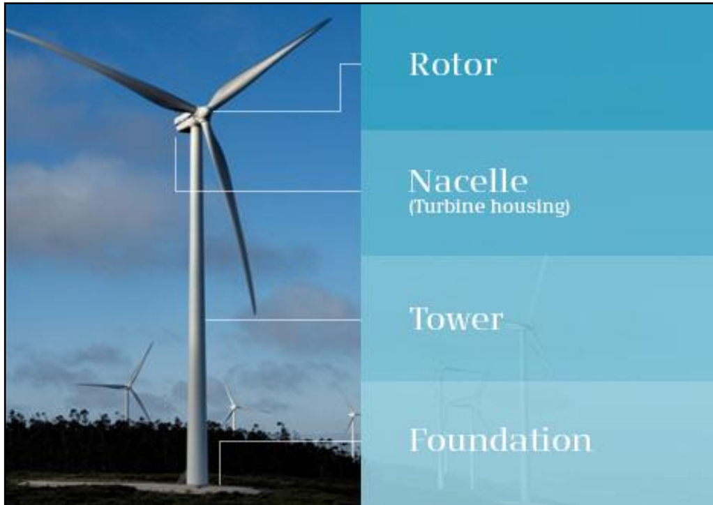
Plate 3-1 Wind Turbine Components.
