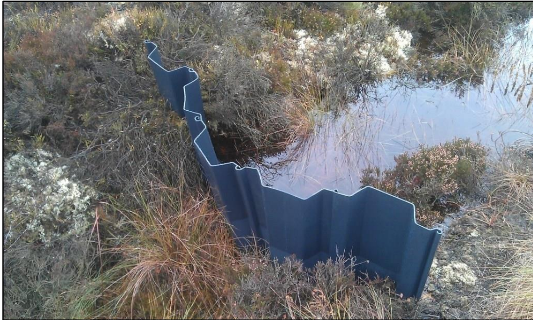
Plate 2.5 Example of plastic dams to be used for on-site drain blocking.
